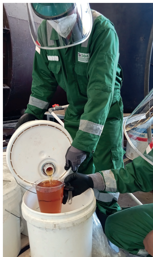
▲ Measuring Corrosion Inhibitor for Hydrotesting. Image courtesy of Tiga Ombak, Cortec® Case History 852.
