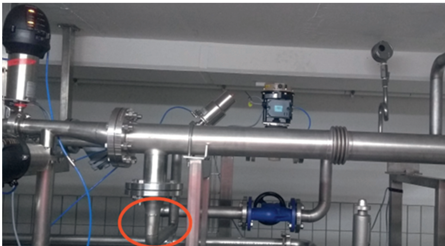
Figure 10. Condensates pipeline with a poor design.
